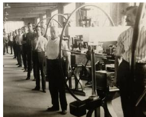
These are siderographers ("transfer men"), craftsmen who either made rolls from hardened dies or made printing plates from hardened rolls. The cylindrical rolls were used to impart design elements like vignettes to printing plates
