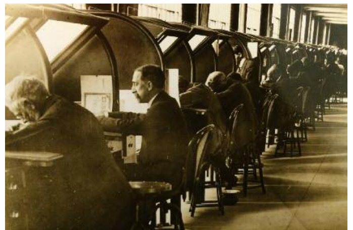
Rows of exclusively male letter gravers are shown hunched over their work under special apparatus for optimizing daylight illumination. These men were responsible for the amazing fine scrip found in bond text
