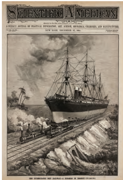
View of ship underway as part of James B. Eads' plan for a 215 kilometer ship railway over the mountain ridge of Tehuantepec in Mexico (Scientific American 1884)
