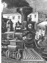
For descriptive purposes, I call these "mushroom" stacks. I suspect the loco on the left was probably burning coal. The loco on the right carries a large spark arrestor and was likely burning wood.
