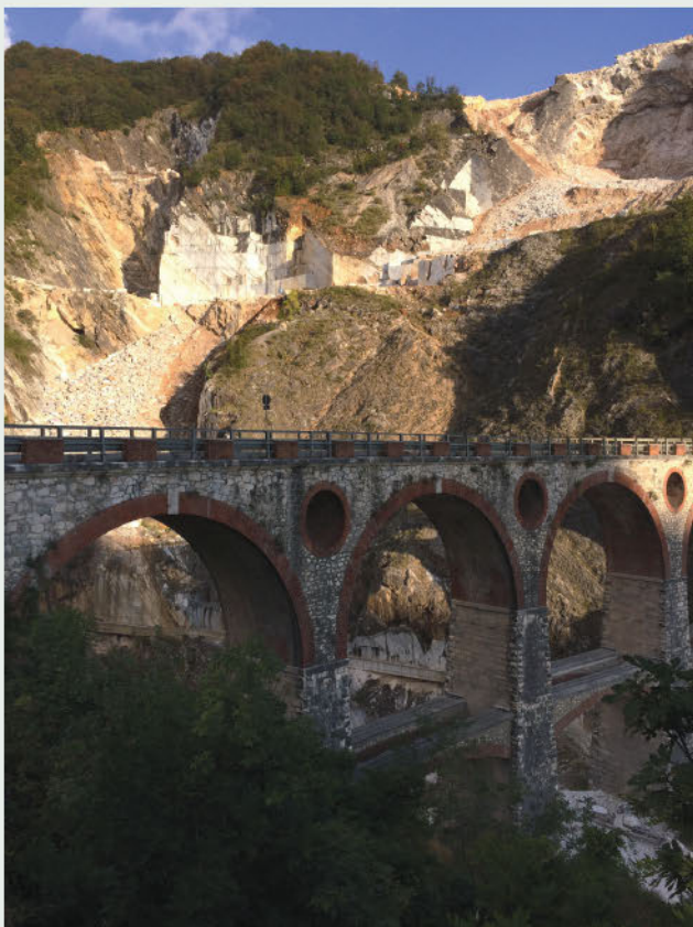
View of railroad viaduct now converted to automotive use, in the background is one of the many quarries still being operated
