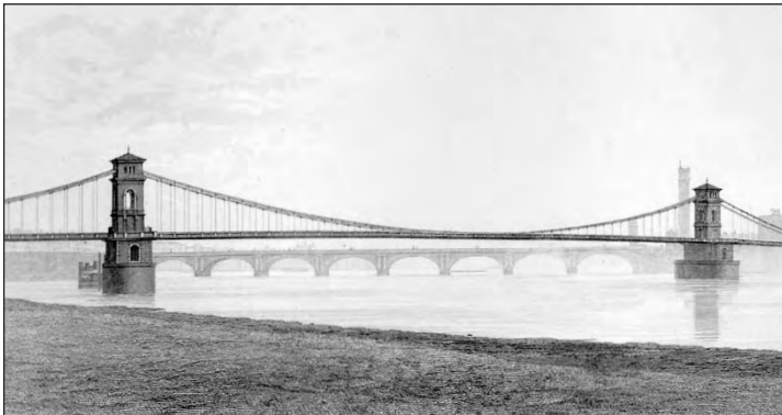
Hungerford Suspension Bridge as built by I K Brunel in 1841-45, showing the chains later re-used for the bridge at Clifton (Bristol), and John Rennie's 1817 Waterloo Bridge beyond
