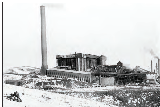
TCC's Copperhill Tennessee smelter looks grim in 1910, but the large boxy building housed the sulfuric acid recovery units that began to reverse the degradation of Basin ecology Courtesy Ducktown Basin Museum
