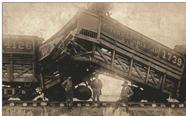
The Street's Western Stable Car Co was a major provider of stock cars to the railroads. This one was wrecked in a washout somewhere in the West
