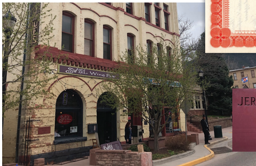
Fig. 4 Jerome Wheeler's bank building in Manitou Springs ca 1890, with cornerstone (inset)
