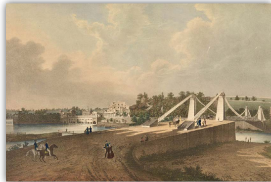
Fig. 2. Hand-colored "View of the Wire Bridge at Fairmount, Philadelphia. Erected in 1842."
