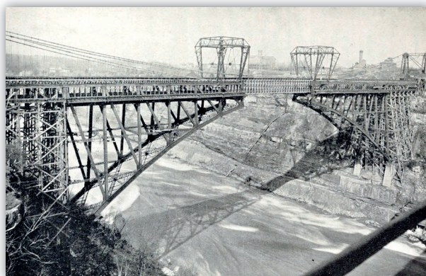
Figure 6. The new Lower Arch Bridge, under construction, surrounds the old Suspension Bridge. (Public Domain)
