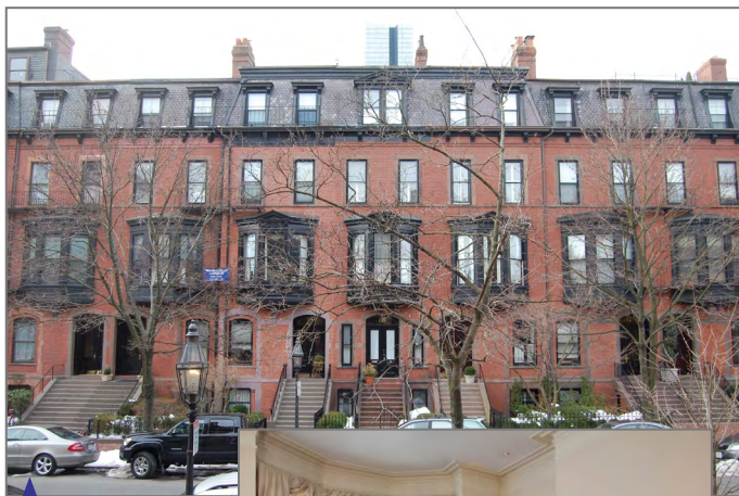
Exterior of 114 – 126 Marlborough St. Boston
