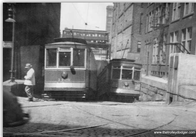
West entrance to the Van Buren St. Tunnel showing trolleys and, up above, the elevated tracks of the Union Station steam railroads. When this photo was taken ca 1920 the line had been electrified
