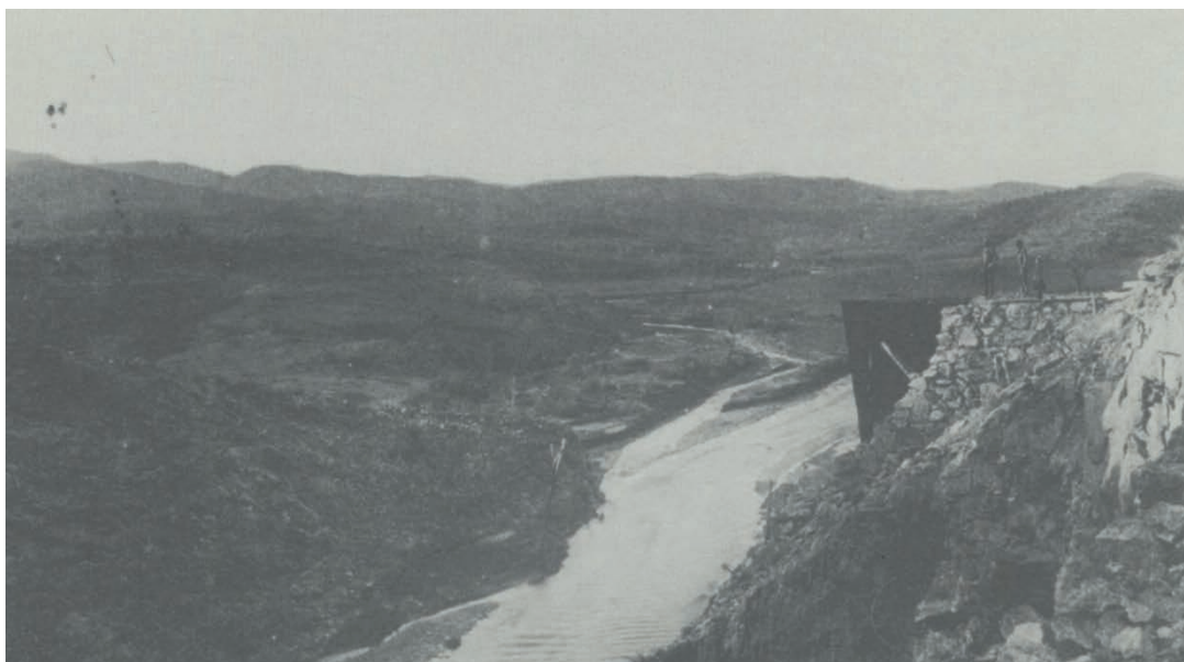
Fig.4. Photo of the site after the dam washed out. A small portion of the dam remains at right
